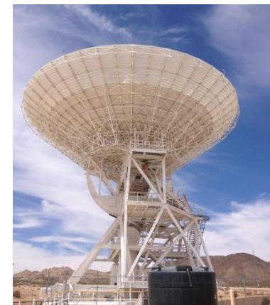
34 m Beam Waveguide
