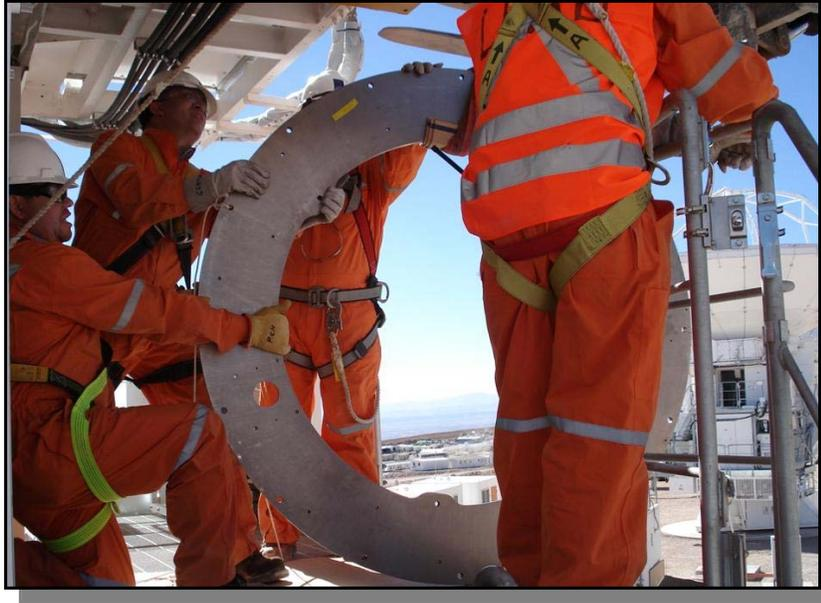
AIV team hoisting the first FE Support Structure into the ACA 12-m antenna.
